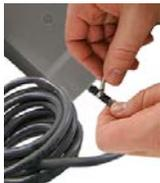
4. Beginning over the installed electrical tape, twist the Itron cable armor onto the remote water module cable using a right-handed twist.
